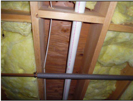
6.5 Item 1(Picture) missing insulation
