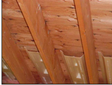
1.5 Item 3(Picture) Soffit Vent
