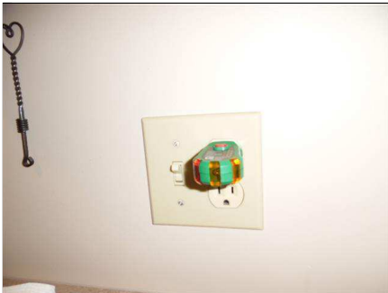
3.8 Item 1(Picture) outlet not working
