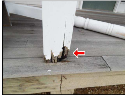
2.3 Item 3(Picture) Post deterioration
