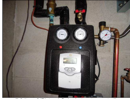
7.2 Item 2(Picture) Solar hot water controller
