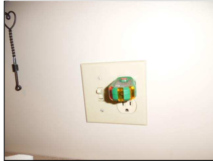
3.8 Item 1(Picture) outlet not working
